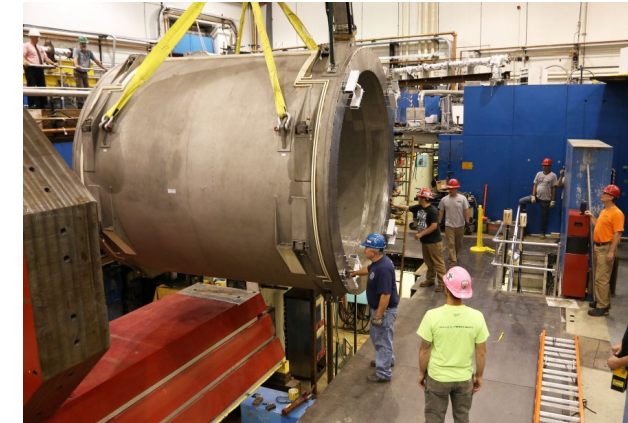
The 26-ton solenoid being removed from L-Zero.
