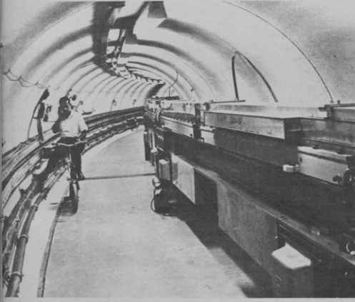
CONSTANT VIGILANCE: Prof. Raphael Littauer, physics, is shown adjusting steering coils which are distributed around the synchrotron ring.
