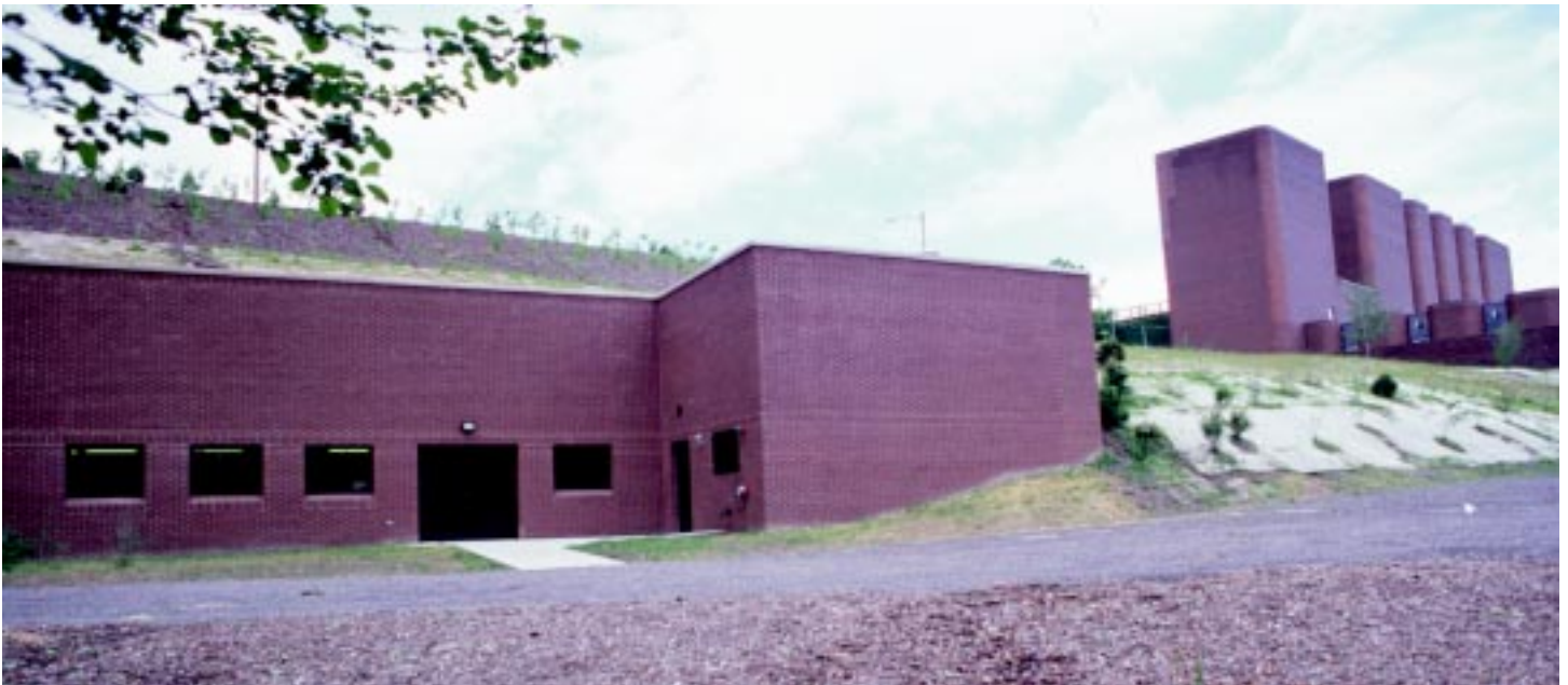
Figure 3: G-line building from the exposed south-facing exterior. The rest of the building is underground. Wilson Laboratory is to the right and the Kite Hill parking lot 50' above the G-line floor level. The storage ring is in a bored tunnel (not shown) 50' under the Kite Hill parking lot. Photo by: Charles Harrington, Cornell University Photography.
