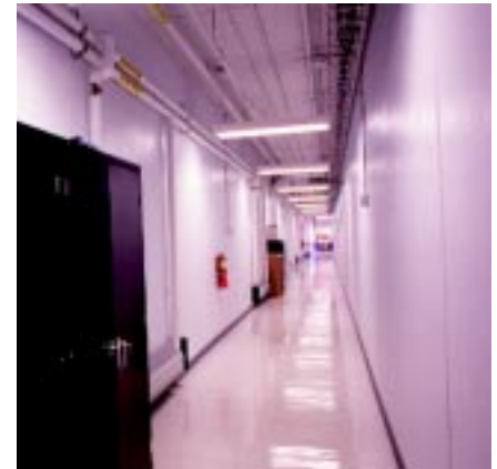
Figure 5: View down the 140' long link tunnel from G-line to Wilson laboratory. This link provides all-weather underground access to G-line for staff and users. Photo by: Charles Harrington, Cornell University Photography.
