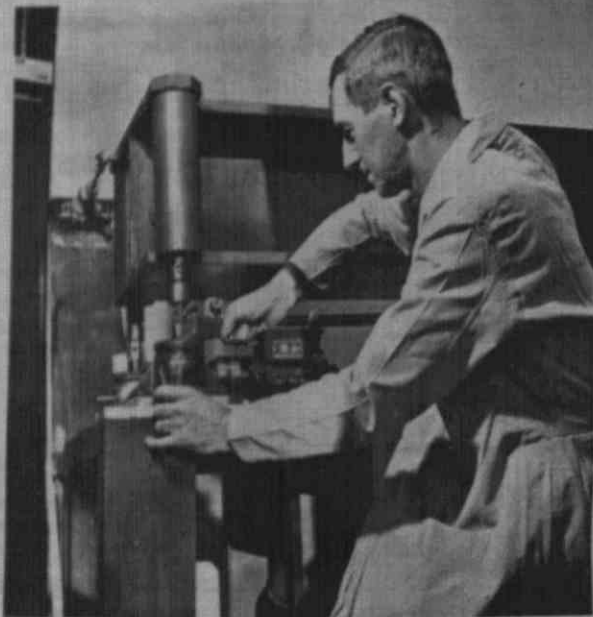
Foreman adjusts one of three jacks which will help maintain alignment of steel girder sections of the accelerator.
