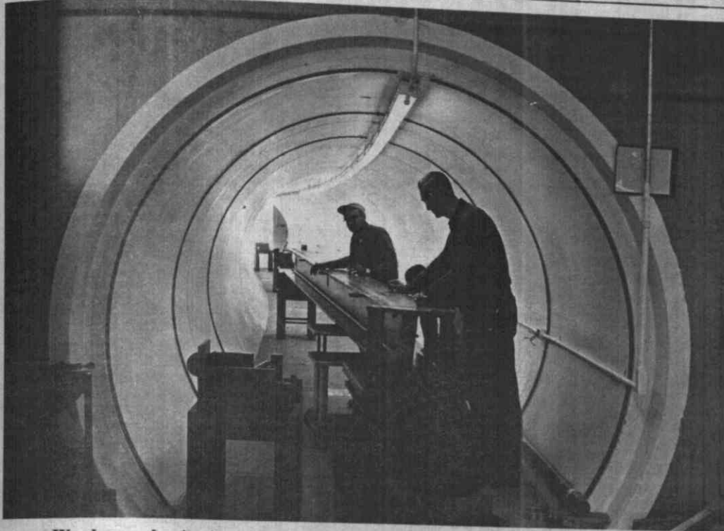
Workmen begin installation of first steel girders in "model" tunnel.
